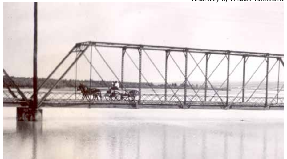
Metal Isleta bridge constructed circa 1931 to replace original wooden bridge. Courtesy of Louise Chewiwi.
